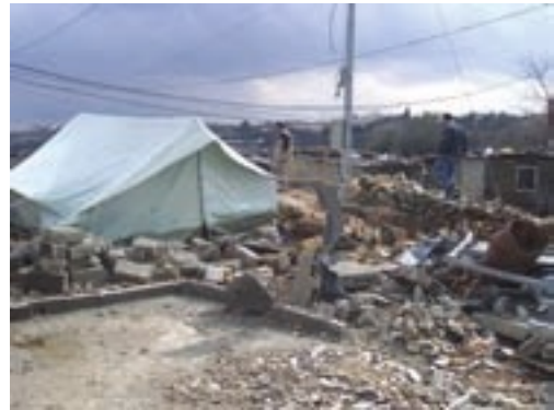
A family forced to live in a tent, amid the ruins of their former home.
